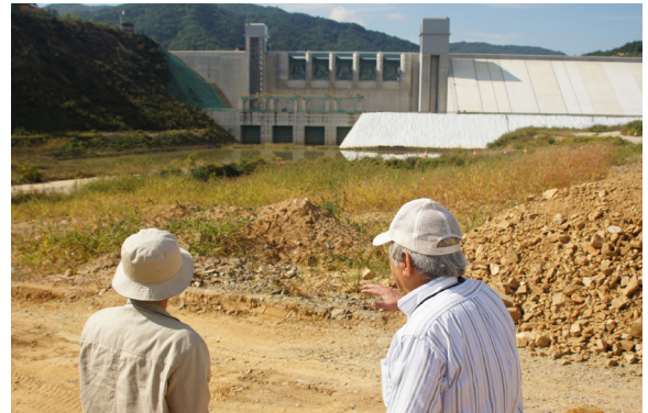
Yeongju dam constructed in the Naesung River. 2014
